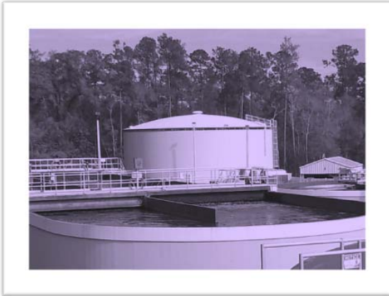
City's Water Reclamation Facility showing the new 1.5 million gallon reclaimed water storage tank.
